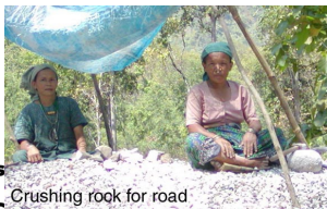
Crushing rock for road
