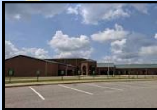
Terrell County SBHC
